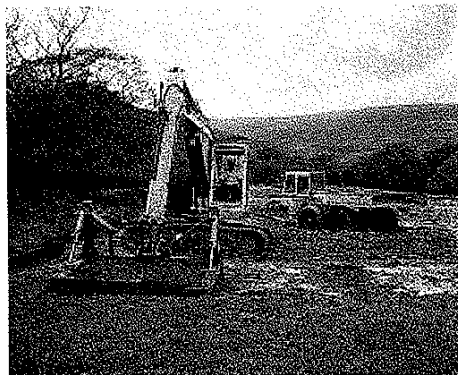
Plate 6.12 Average sized turves (2.35 m x 1.3 m) using macro-turfing machinery
