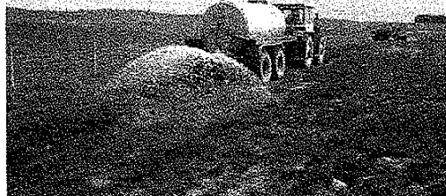
Plate 6.30 Watering replaced heather turves after a pipeline installation at Lazonby, Cumbria
