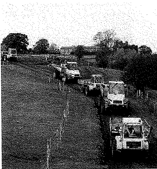
Plate 6.16 Flatbed dump trucks moving grassland turves at Manchester Airport
